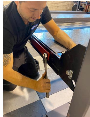
16. Bolt the ramp and the flat bars for the drive-up ramps.
